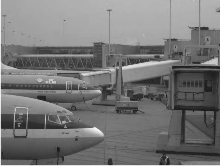
Figure 9.6 Pier D at Schiphol. Note the horizontal division produced by the new top level in order to divide Schengen passengers from others. Photo courtesy of author.
